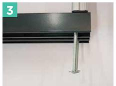
Screw through the pre drilled holes in frame into the low threshold securing them both together.
