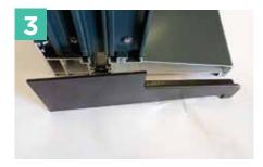
Silicone seal the end of the cill and attached the end caps to the cill to create a water tight joint.
