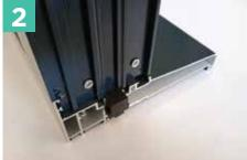
Insert the bung into the top part of the cill between the cill and frame.
